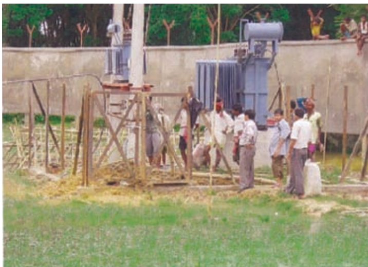
Installation of transformer for drawing construction power
