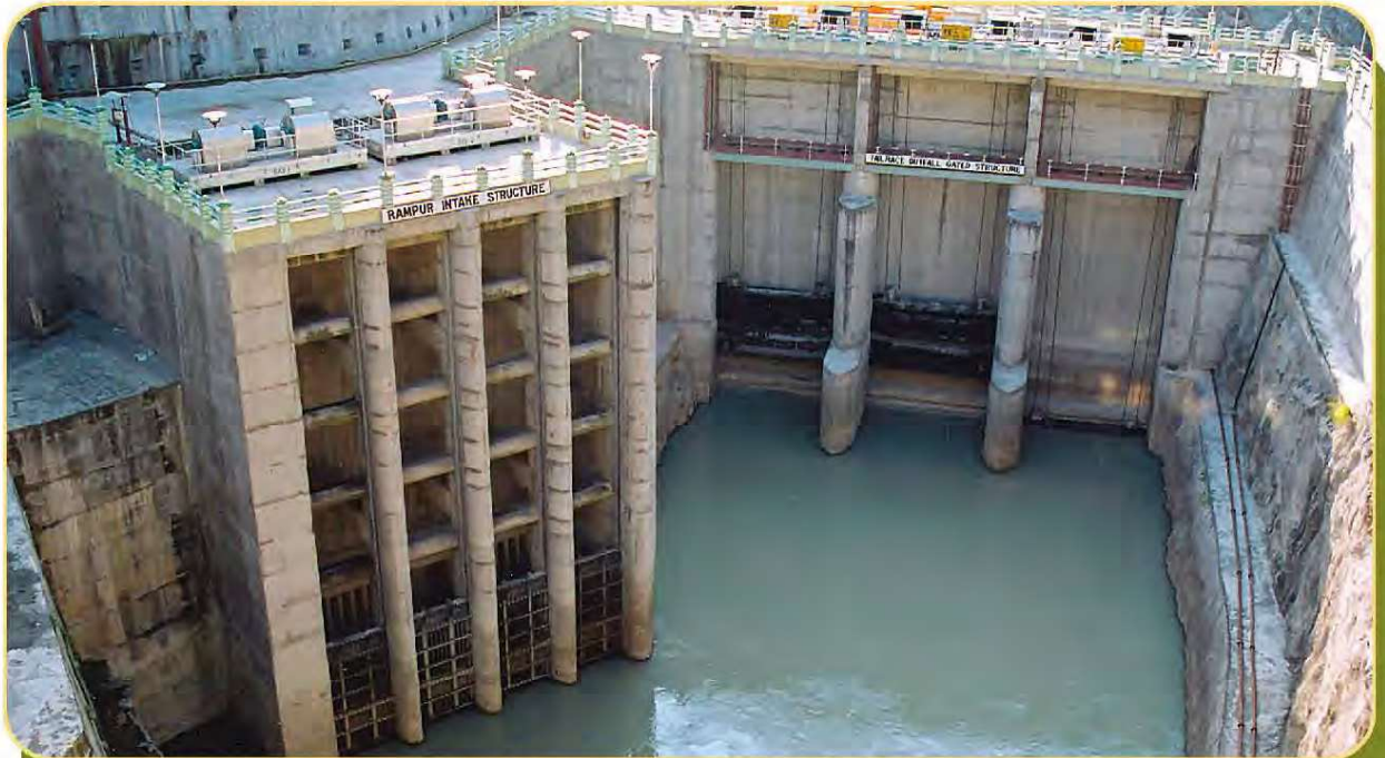
Intake Structure of 412 MW Rampur H.E. Project of SJVNL in Himachal Pradesh
