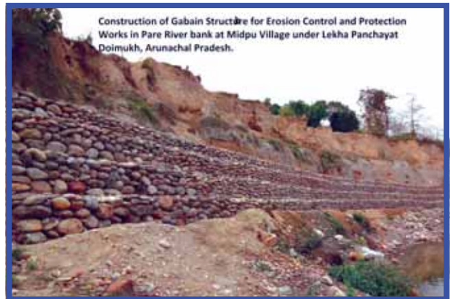
Construction of Gabion Structure at Arunachal Pradesh
