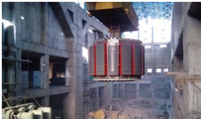
Lowering of Rotor, Unit III on 28 th February 2017
