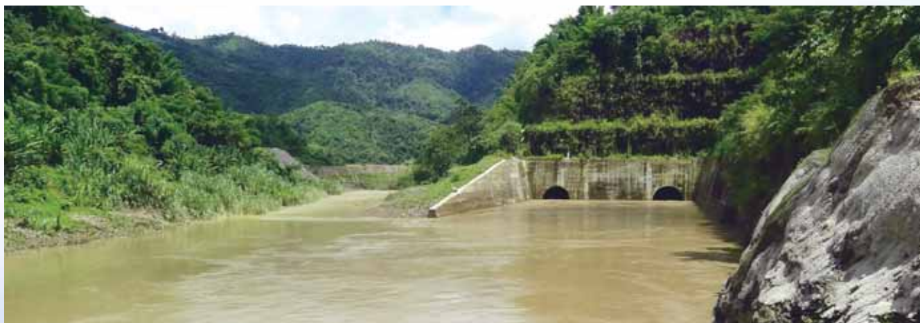
Downstream Cofferdam, Tuirial Hydro Electric Project
